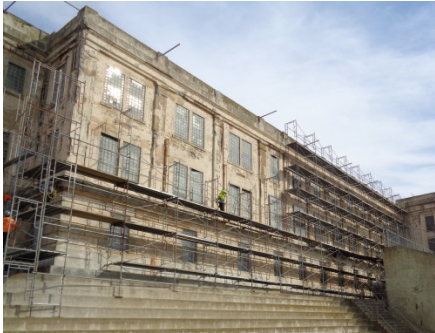
Cellhouse exterior being readied for repair.
